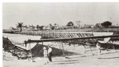
Fig. 1.8 A view from the south of the Shuman Boys solar collector system constructed at Maadi, Egypt, in 1913.
